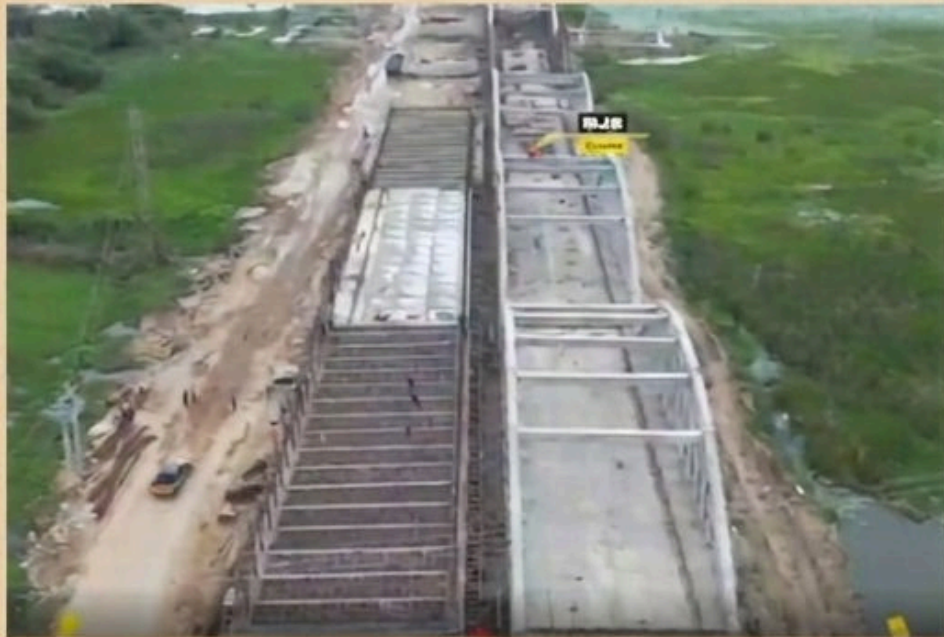
RCC Bow String Major Bridge construction work under progress
