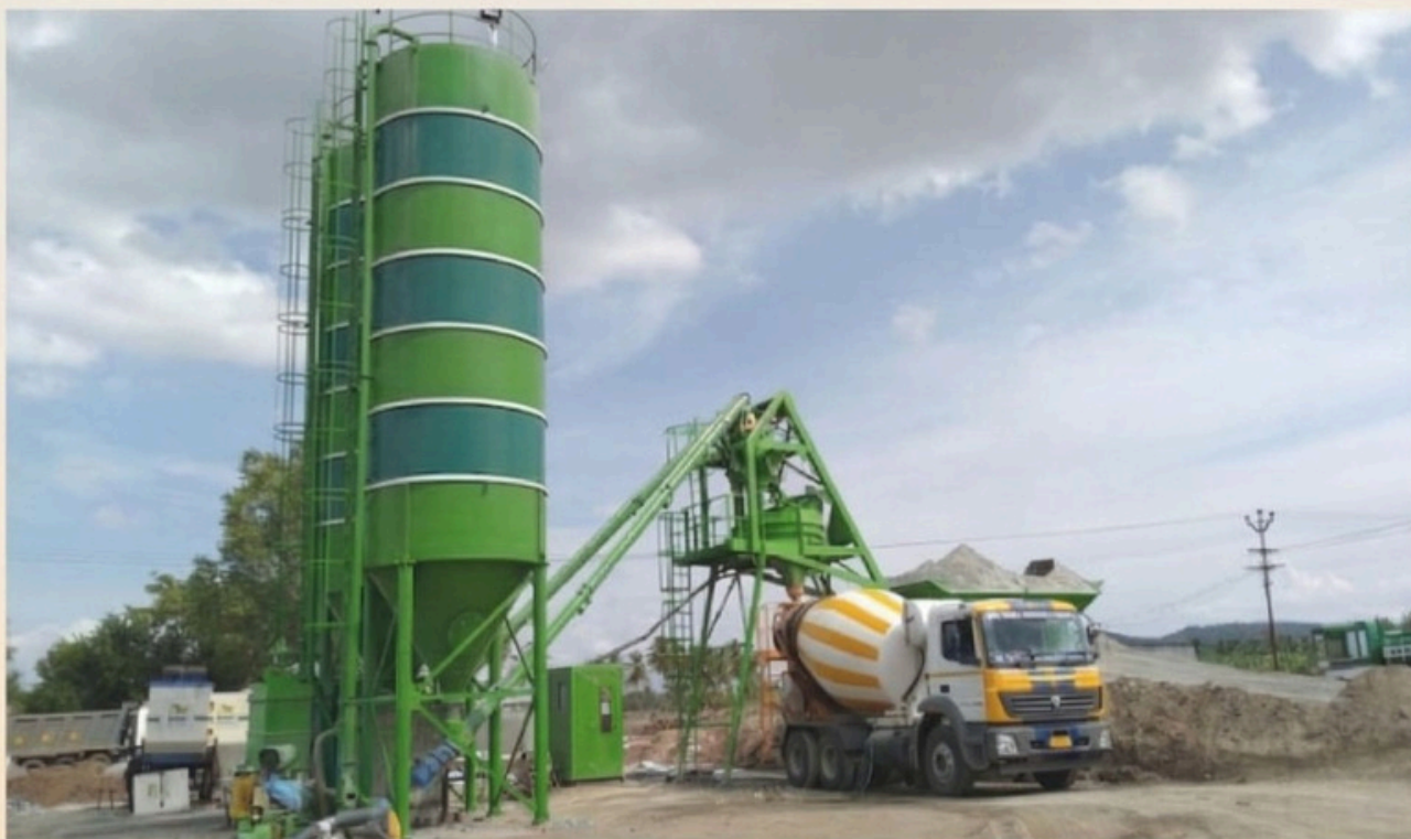
Ready Mix Concrete Plant CP-30 & M1
