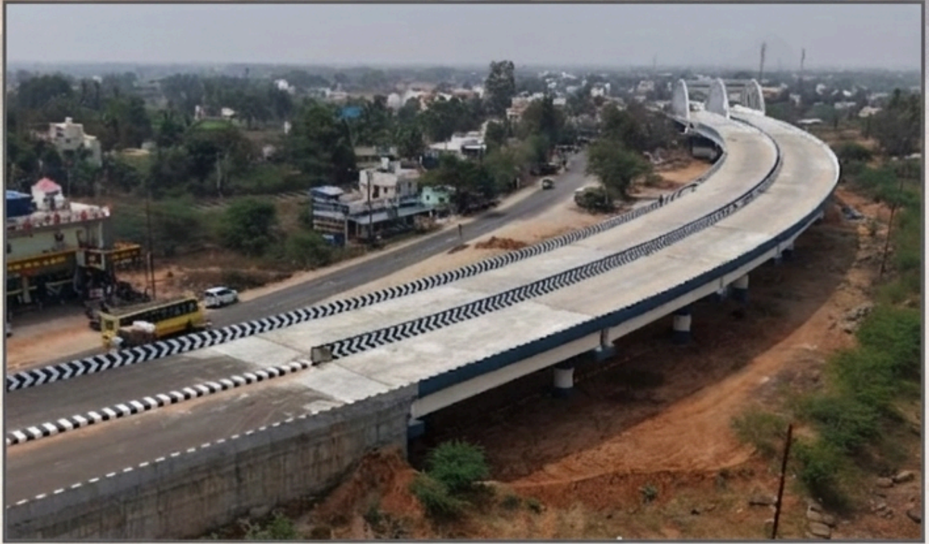
Aerial view of Major Bridge with ROB
