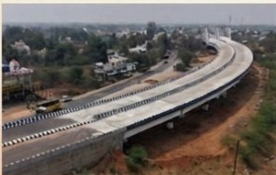
ROB with Bow String Steel Girder (Span 1 X 51.40m X 2)
