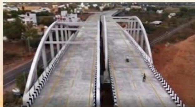
ROB with Bow String Steel Girder (Span 1 X 51.40m X 2)
