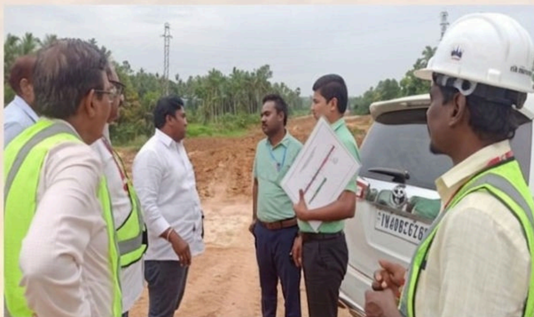
SITE VISIT CONDUCTED BY THE REGIONAL OFFICER, NHAI, MADURAI IN PROJECT OF FOUR LANING OF LEFT-OVER WORKS INCLUDING ADDITIONAL STRUCTURES IN KERALA / TAMIL NADU BORDER - KANYAKUMARI (NH 47) AT NAGERCOIL
