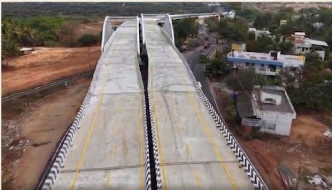
ROB with Bow String Steel Girder (Span 1 X 51.40m X 2)
