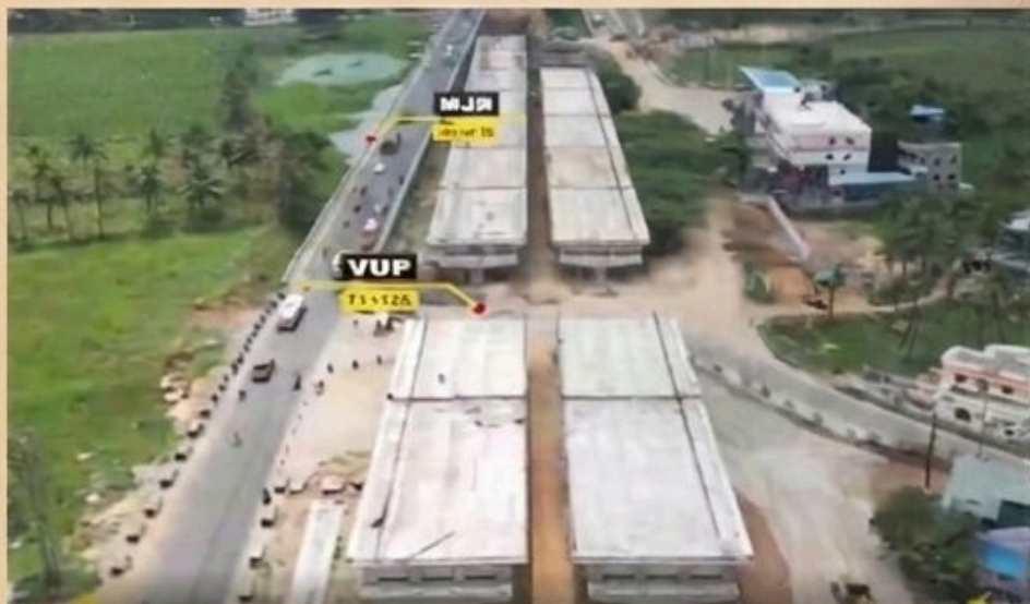
Major bridge cum VUP construction work under progress.
