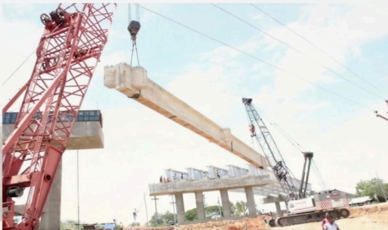
Road Over Bridge in Lieu of Exg. LC No. 201 at KM: 271/0-1 between Ariyalur and Sillakkudi Stations. Composite Girder - 1 X 44.0m and PSC I Girder - 2 X 31.0m
