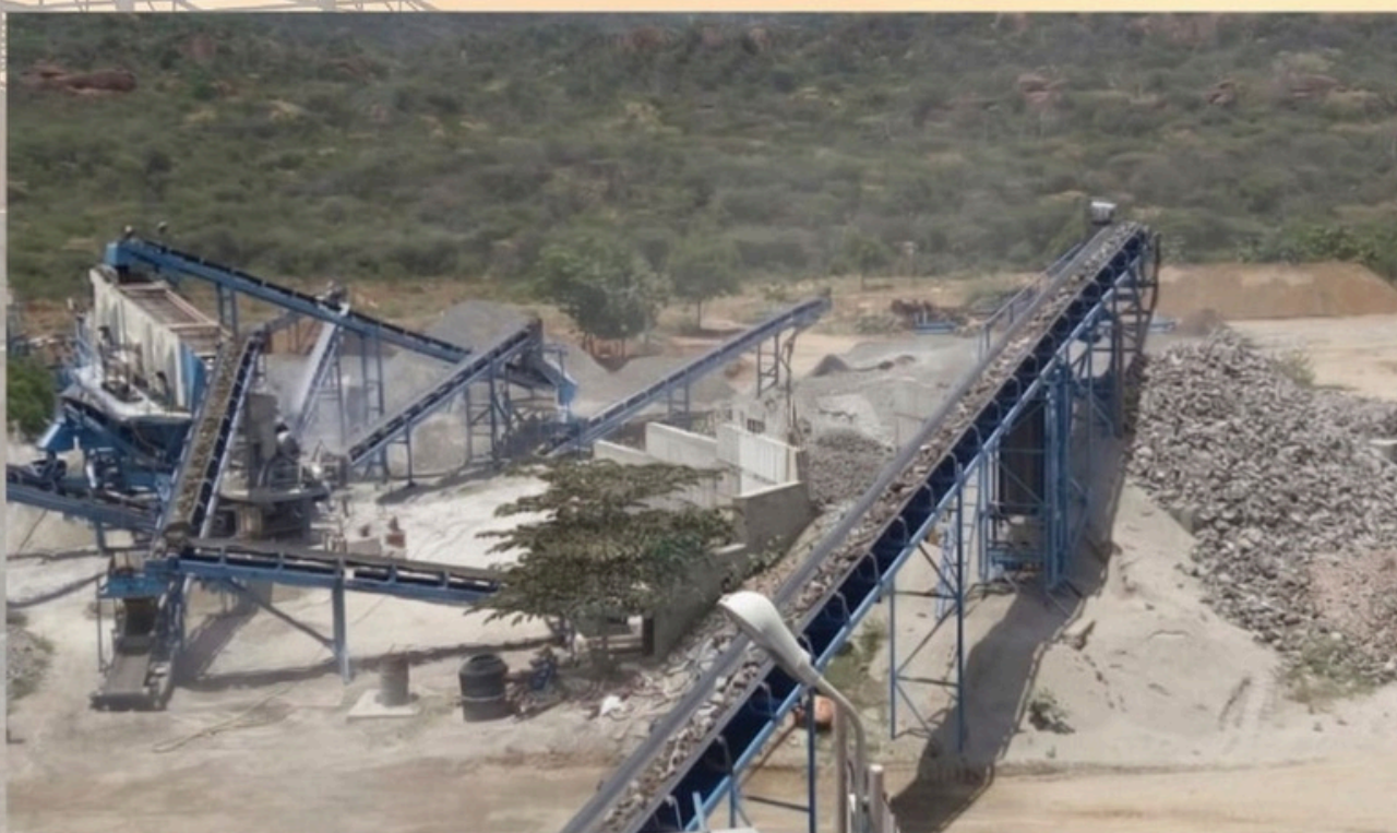
VSI Crusher at Andipatti, Theni
