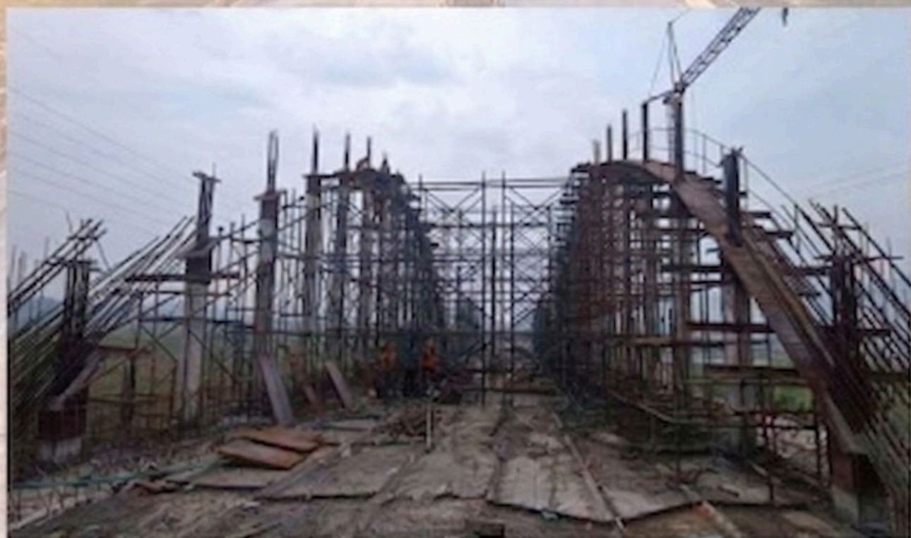
Ch 79+642 Major Bridge RHS Span No.2 Bow bottom staging work
