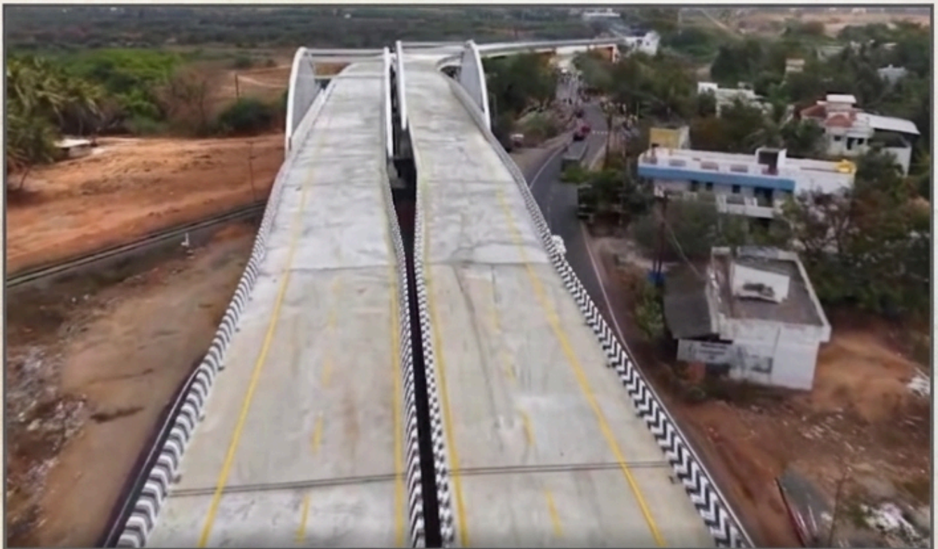
View of Bow String Steel Girder (1 X 51.40 X 2)
