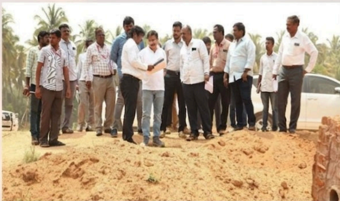
SITE VISIT CONDUCTED BY THE REGIONAL OFFICER, NHAI, MADURAI IN DINDIGUL - THENI - KUMILI (NH 183) PROJECT
