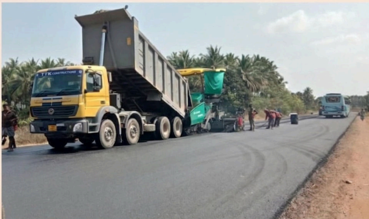
DINDIGUL-THENI-KUMILI NH OVERLAYING
