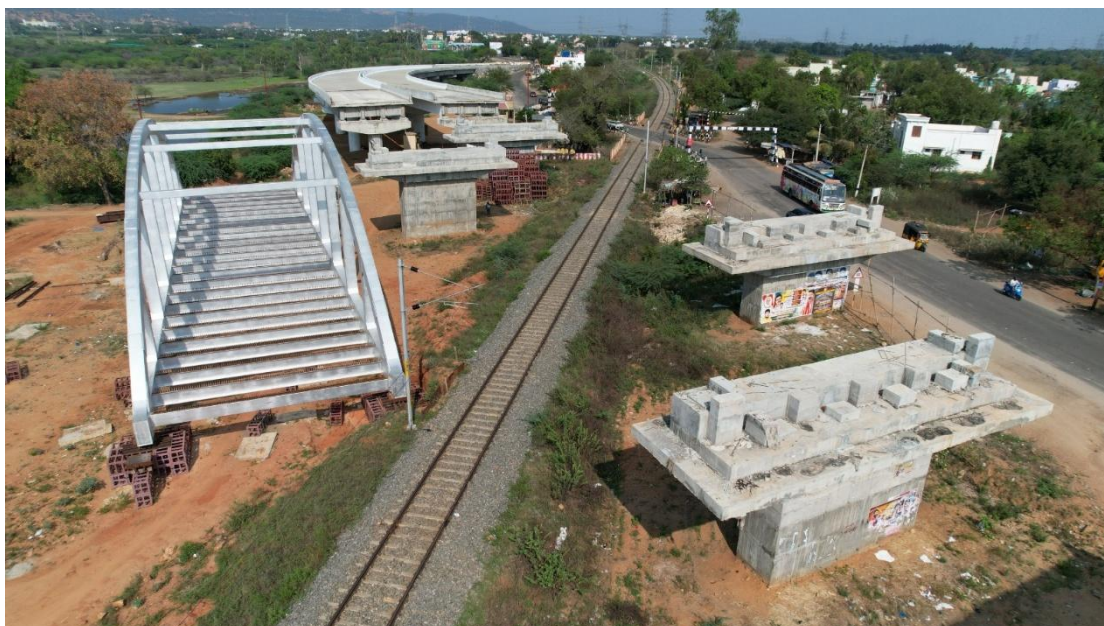
Construction of Major railway ROB bridge @ LC No.17 (Span 1 X 51.4m) between Vadapalanji and Usilampatti Railway Station on Madurai – Cochin section of NH 49 Extn.
