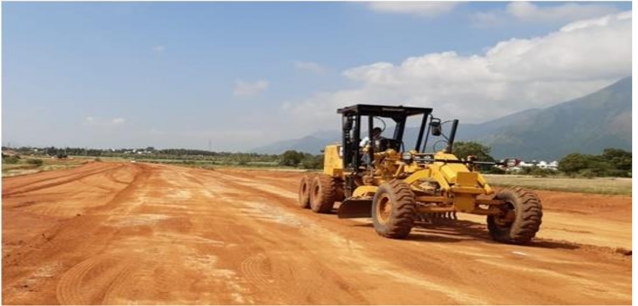
Embankment Grading
